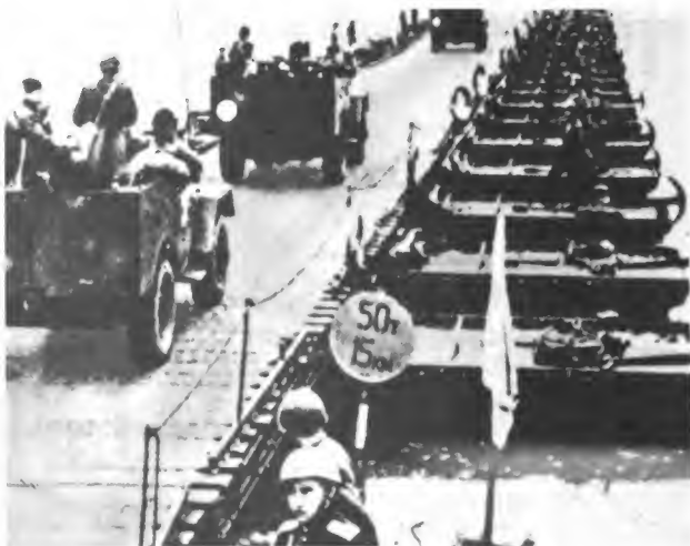
Figure 6-49. Ponton bridges. Light and heavy-weight ponton bridges are employed by the Soviet Ground Forces. The LPP light ponton bridge (above) can carry up to 40 tons, and the heavy TPP (below) carries up to 70 tons. Each ponton is carried on a single truck.
